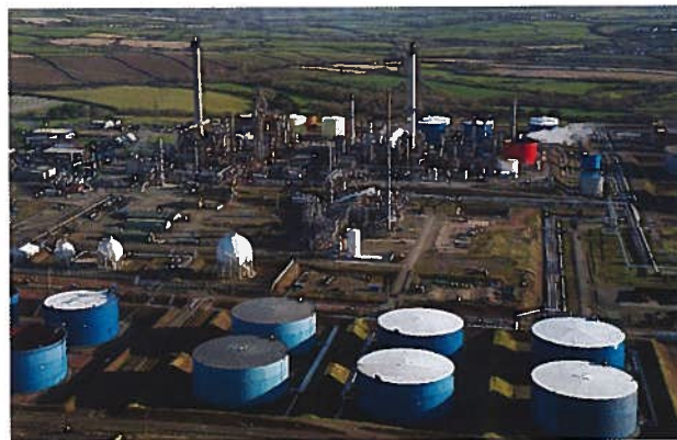
Milford Haven refinery
