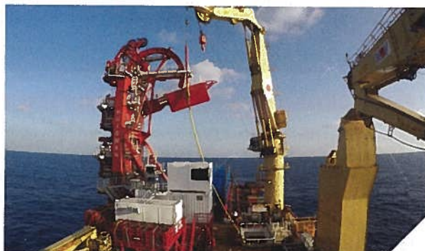
Installation operations at West Nile Delta. Photo from BP.
